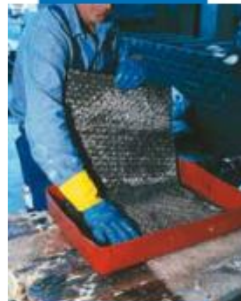
Manual impregnation of MapeWrap C
