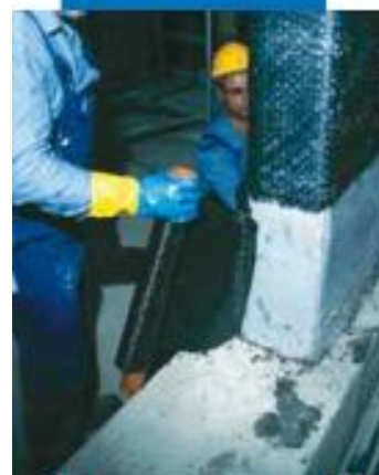
Application of MapeWrap onto the reinforced concrete element
